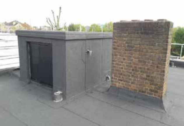
Old Market Square roof
